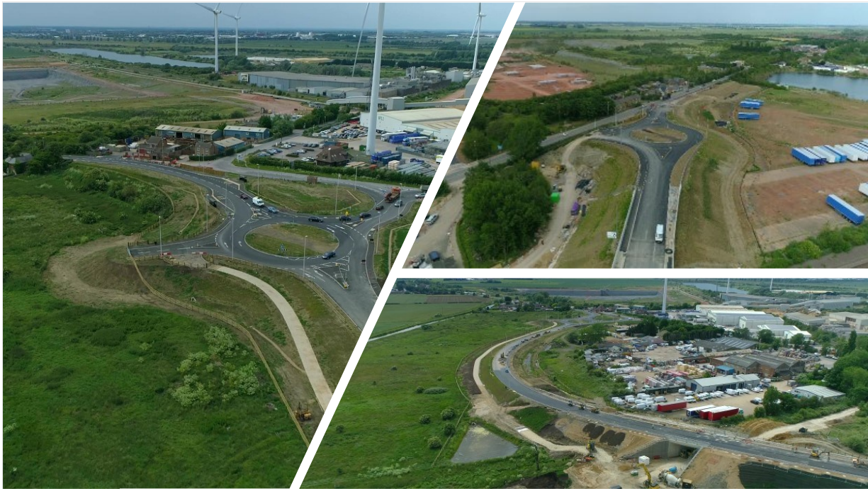
Left, Western Roundabout, Right, Eastern Roundabout, Bottom, section 1 and underpass
