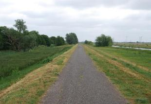
The remainder of the route is in reasonable condition. It shows some evidence of subsidence, likely caused by vehicles, but no major action is currently needed.
