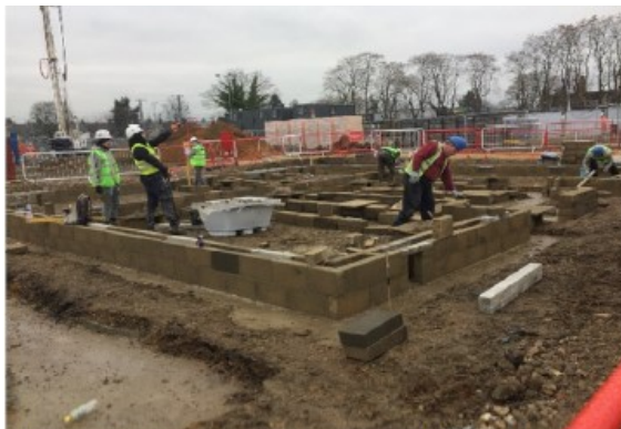
Postal 161 & 162 - Substructure blockwork started
