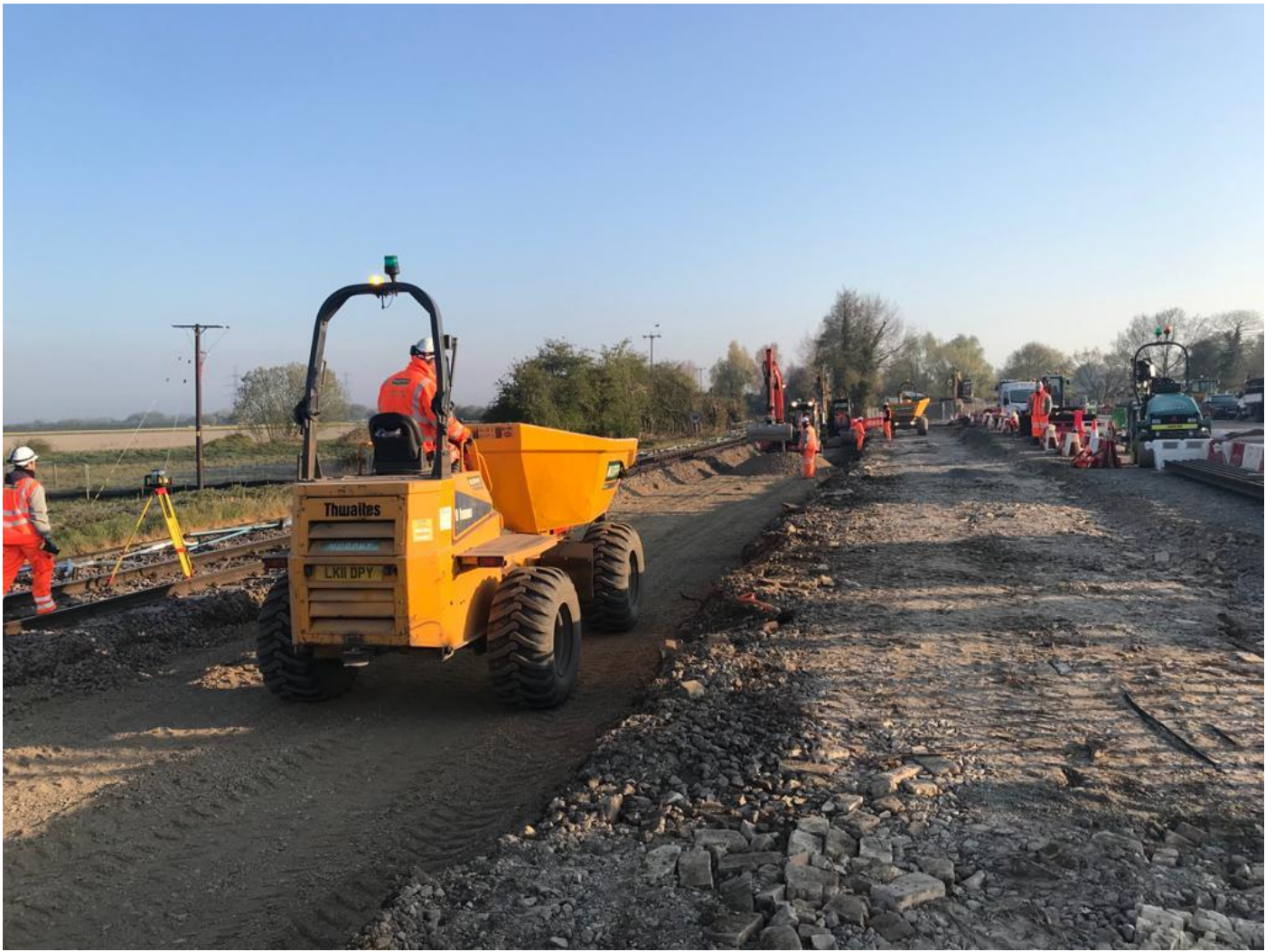
Improving ground for relocated track and platform.
