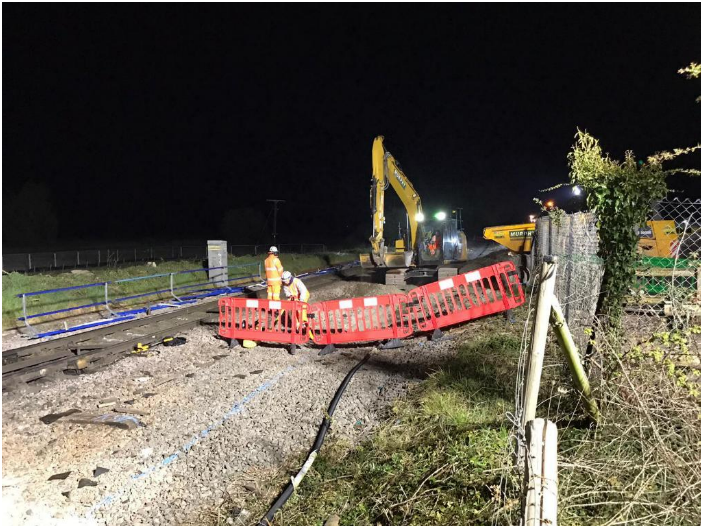
Preparing track to be moved.
