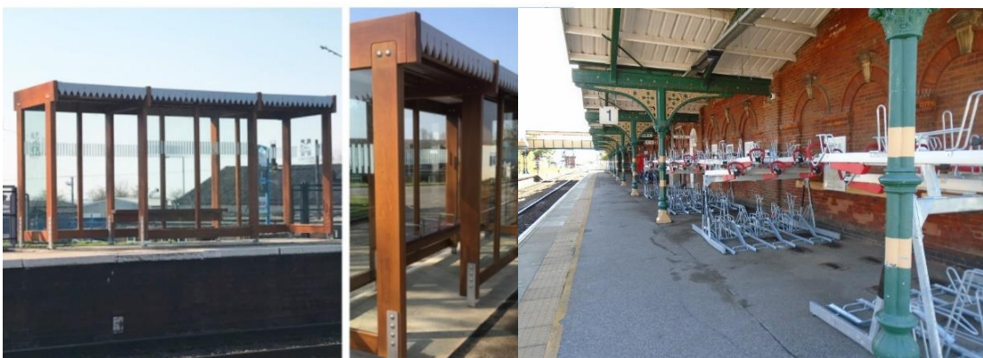
Figure 1: Station Improvements – Waiting Shelter and Cycle Parking
