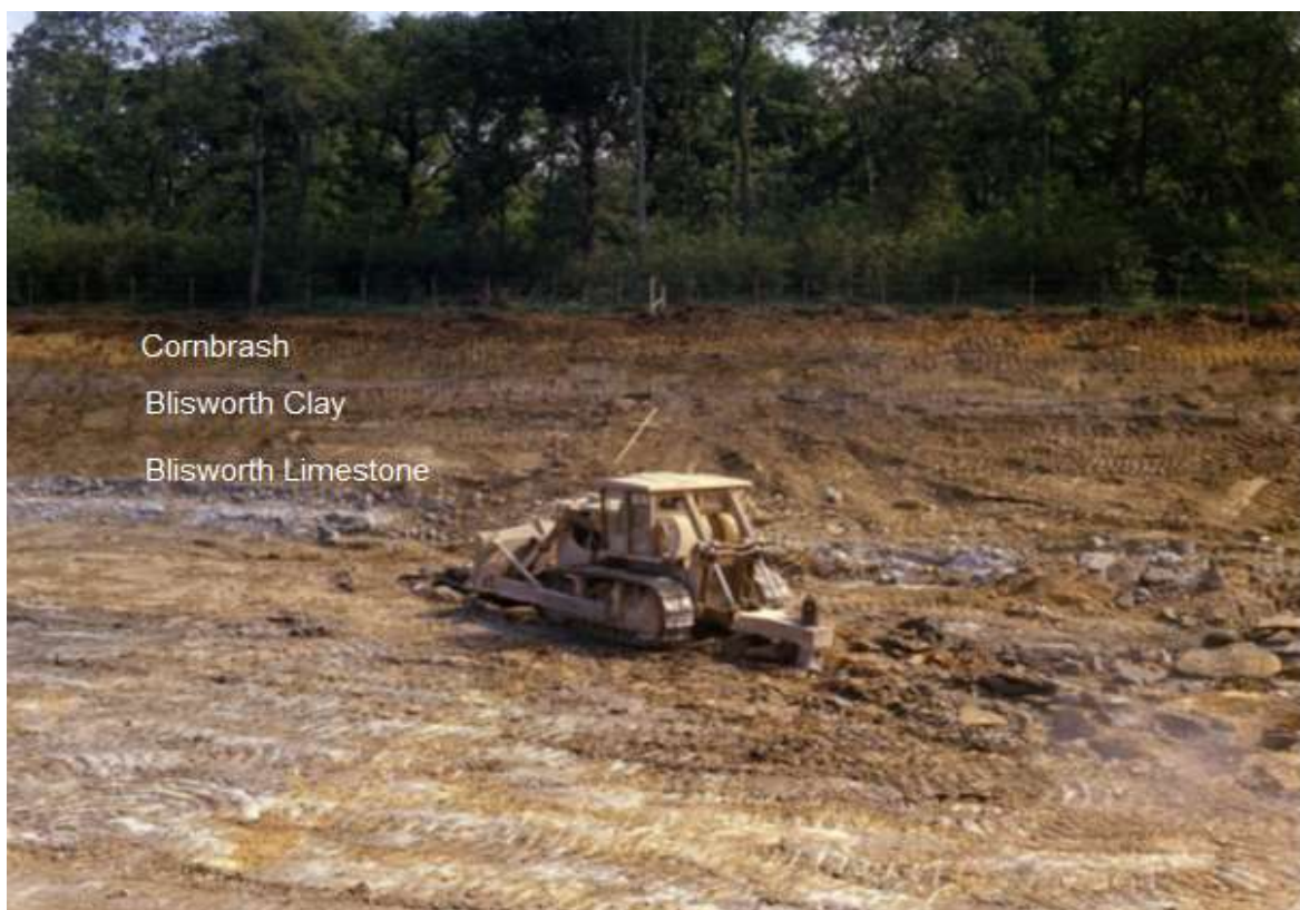
Figure 2.18: Geological Profile During the 1972 A1260 Nene Parkway Construction
