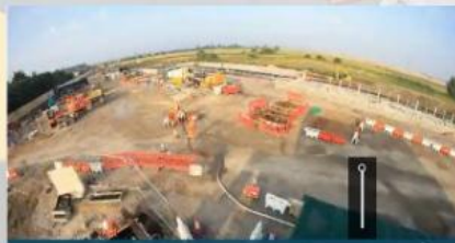
Soham Station construction timelapse
