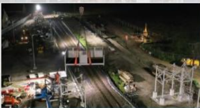
Soham Station Footbridge installation video
