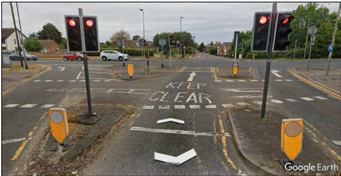
Figure 2.8: View of Northbound Approach to Junction 7, Showing Poor Cycle Provision Crossing Traffic Lanes (Google, 2022).
