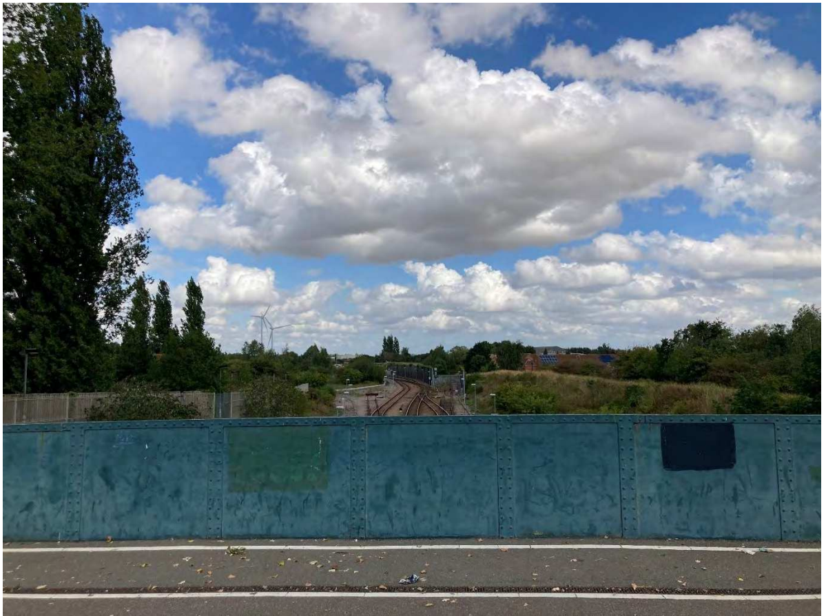
Figure 4-10: Bridge over the railway on Norwood Road (looking north).
