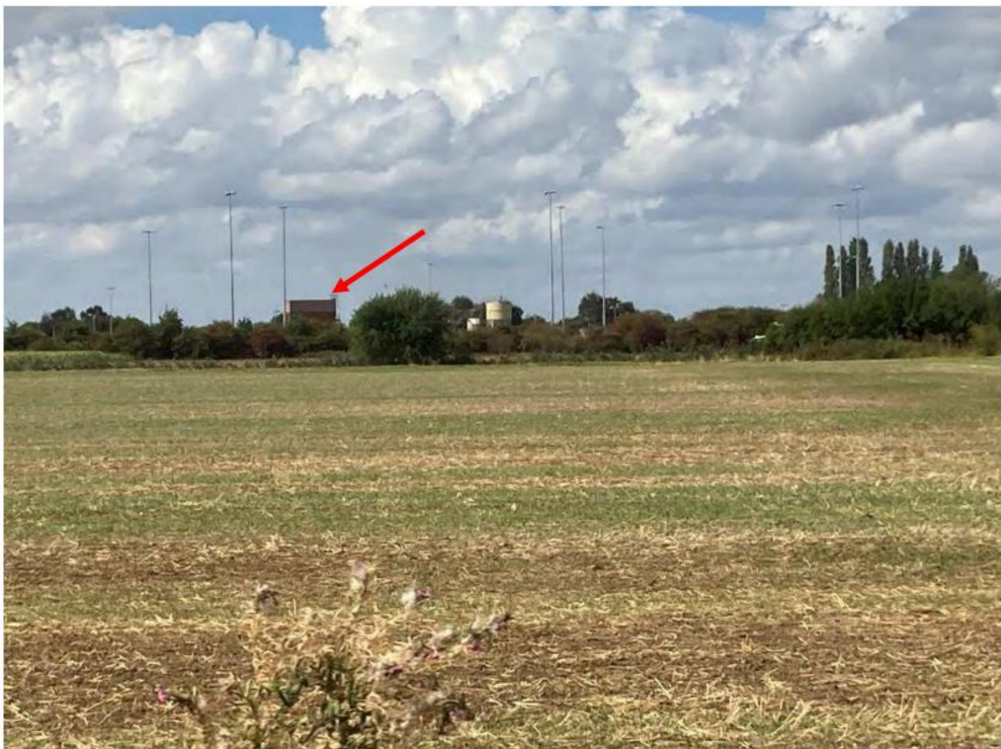
Figure 6-2: View westwards of the water tower (rectangular structure) from Elm Road.
