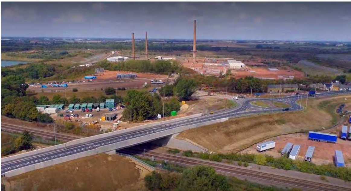
Figure 6.2: Kings Dyke (Source: Jones Brothers)
