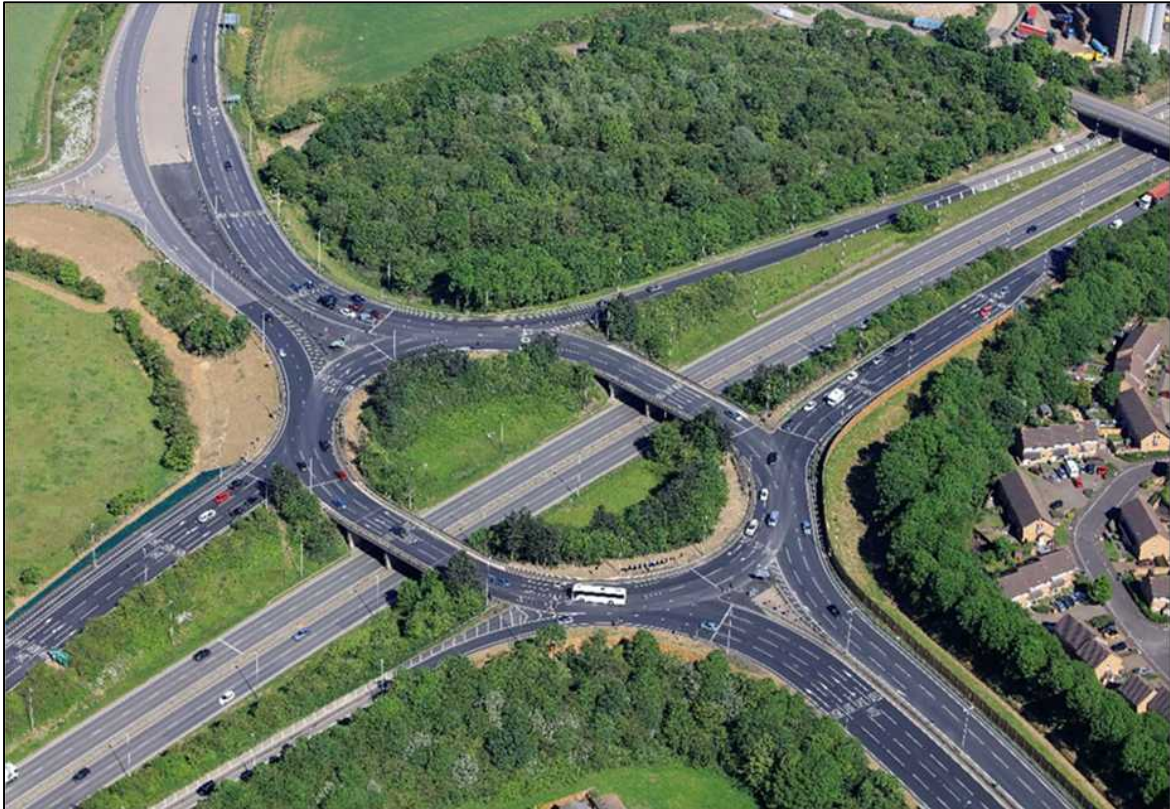
Figure 6.1: Junction 20 Improvement (Post Completion)
