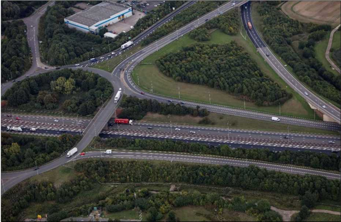
Figure 6.2: Junction 17 (A1M) Improvement (Post Completion)
