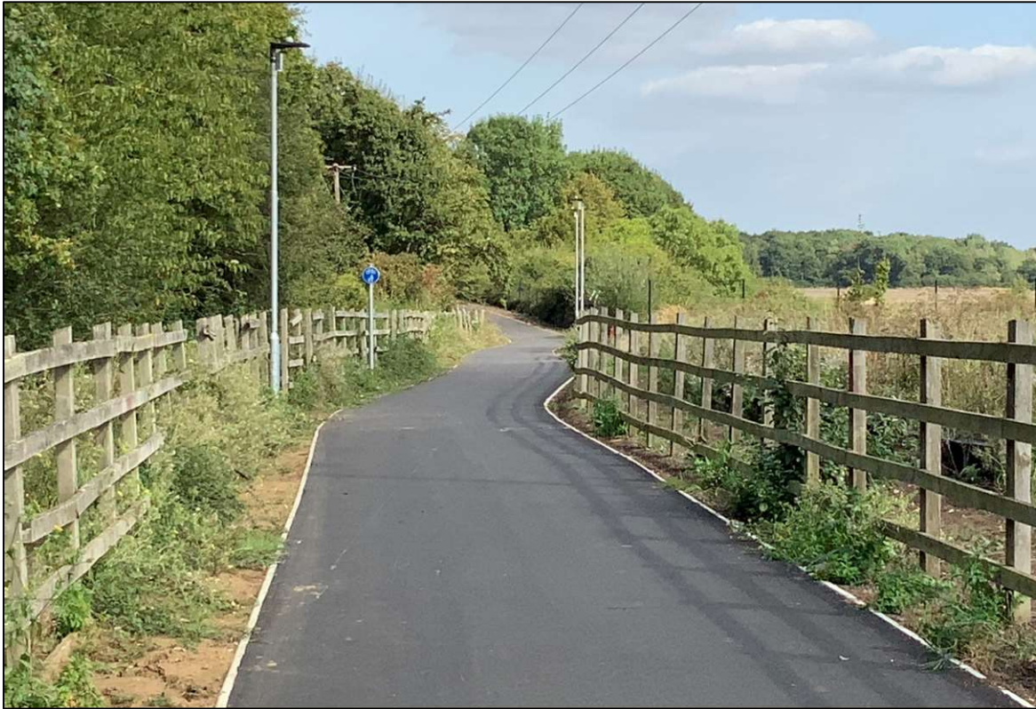
Figure 6.3: Haddon Cycleway Improvement
