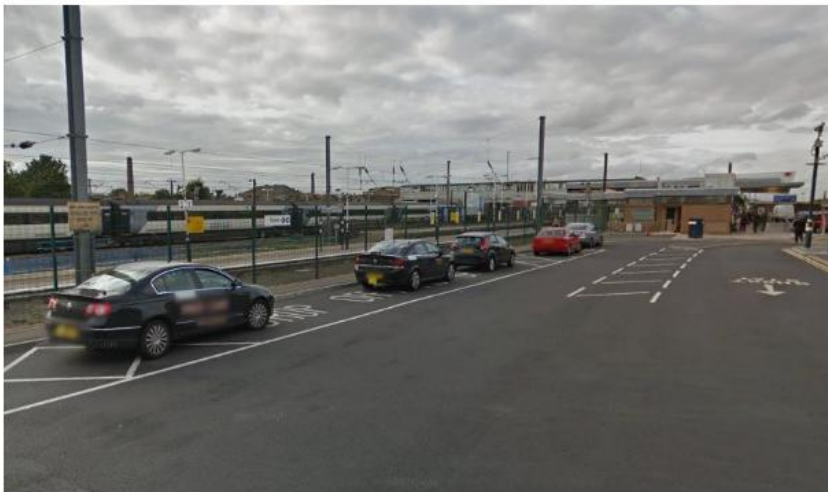
Figure 2.21: Drop-off Zone to the South of the Station Building
