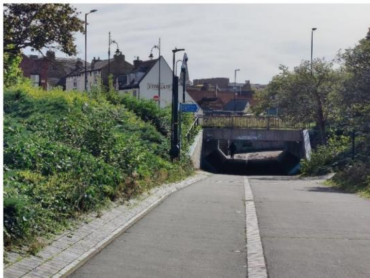
Figure 2.44: Walking and Cycling Path in Queensgate Roundabout
