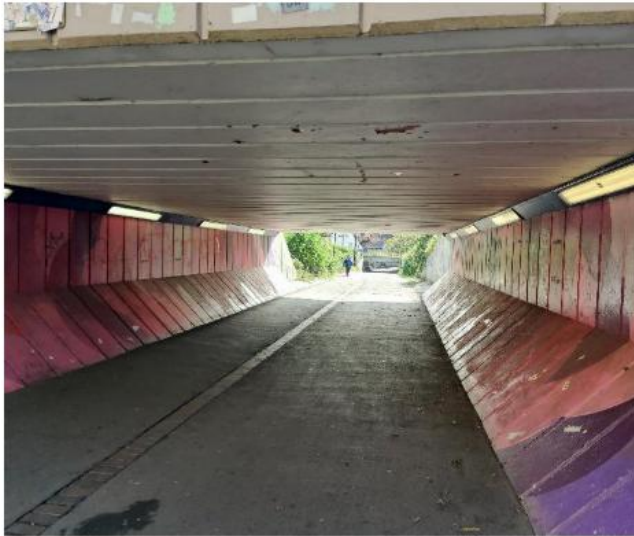
Figure 2.14: Underpass from Station to Queensgate Roundabout
