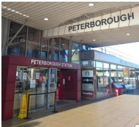
Figure 2.25: Peterborough Station Entrance
