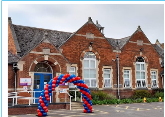
Cambridgeshire Skills deliver adult education at various venues including the refurbished March Community Centre in Fenland. A £400k capital grant from CPCA supported the refurbishments to create a safe and welcoming learning environment.
