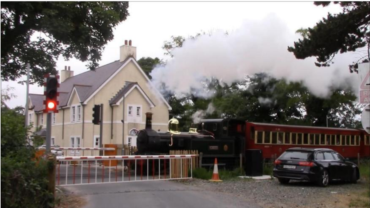
Figure 20 – Simplified Light Rail Barrier Crossing on Isle of Man Steam Railway (Source: YouTube/Perryd Pelle)
