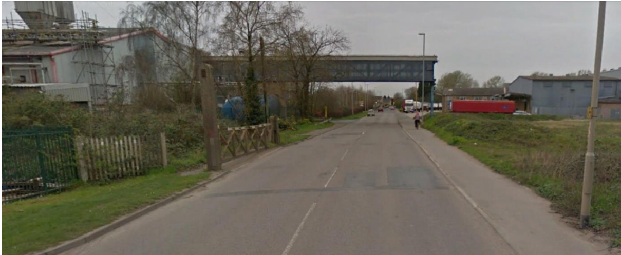
Figure AB14 – Looking West along Weasenham Lane
