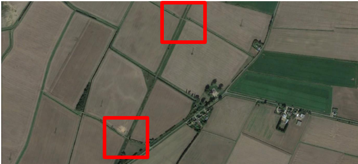
Figure AB20 – Unnamed User Worked Crossings Site Overview
