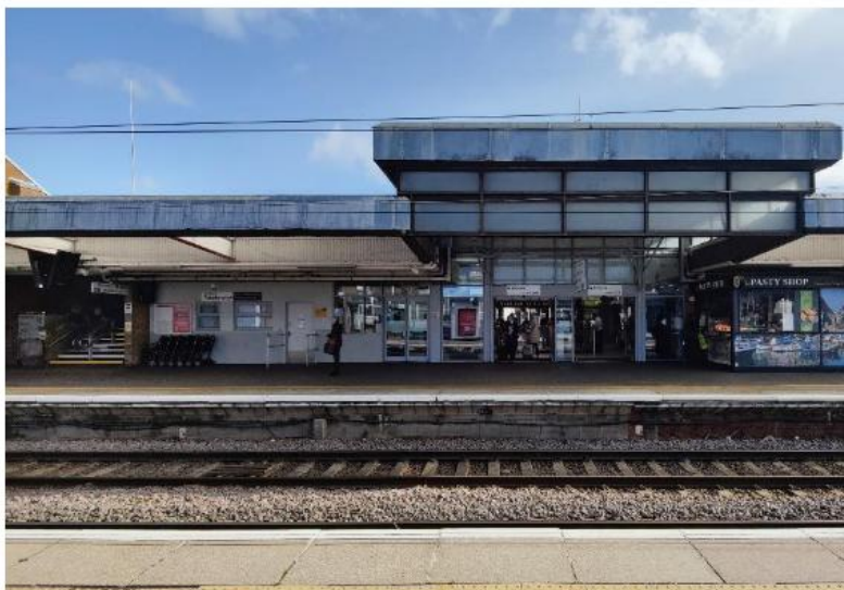
Figure 2.46: Station Entrance on Platform 1
