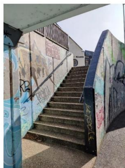
Figure 2.45: Stairs from Crescent Bridge Subway East Underpass
