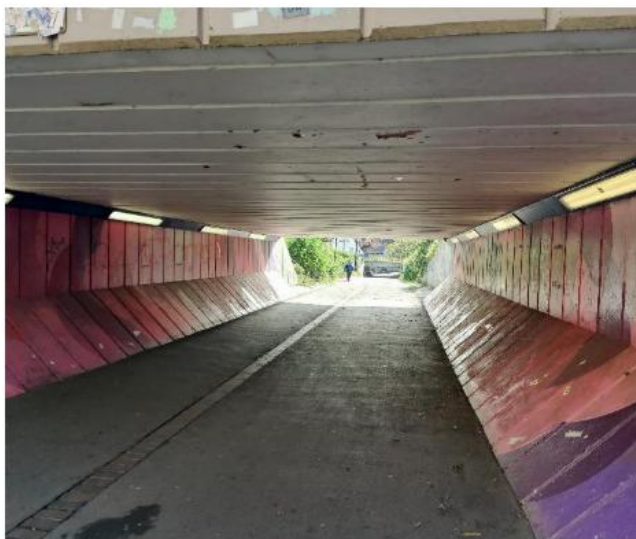
Figure 2.14: Underpass from Station to Queensgate Roundabout
