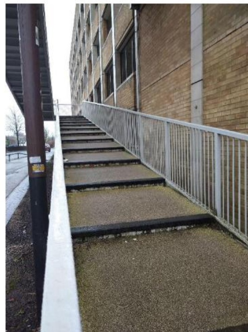
Figure 2.17: Stair Access on Pedestrian Footbridge to Queensgate Shopping Centre
