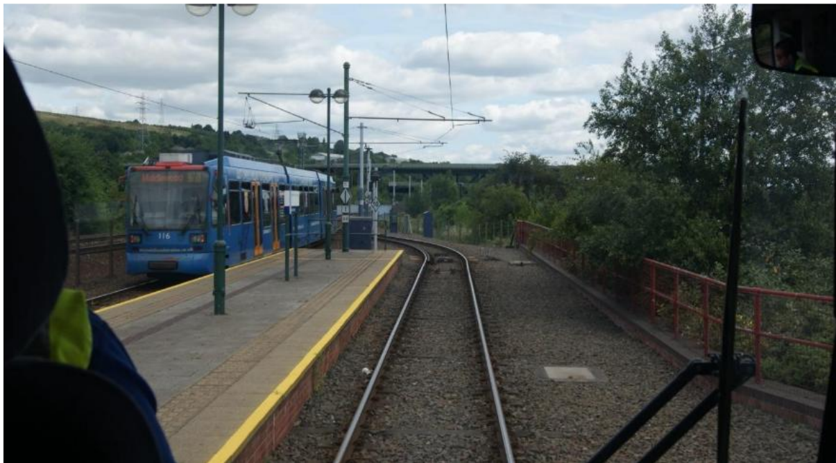
Figure 14 – Example Single Line Occupation Tramway Controls at Meadowhall Interchange, Sheffield (Source: Ian Ambrose)
