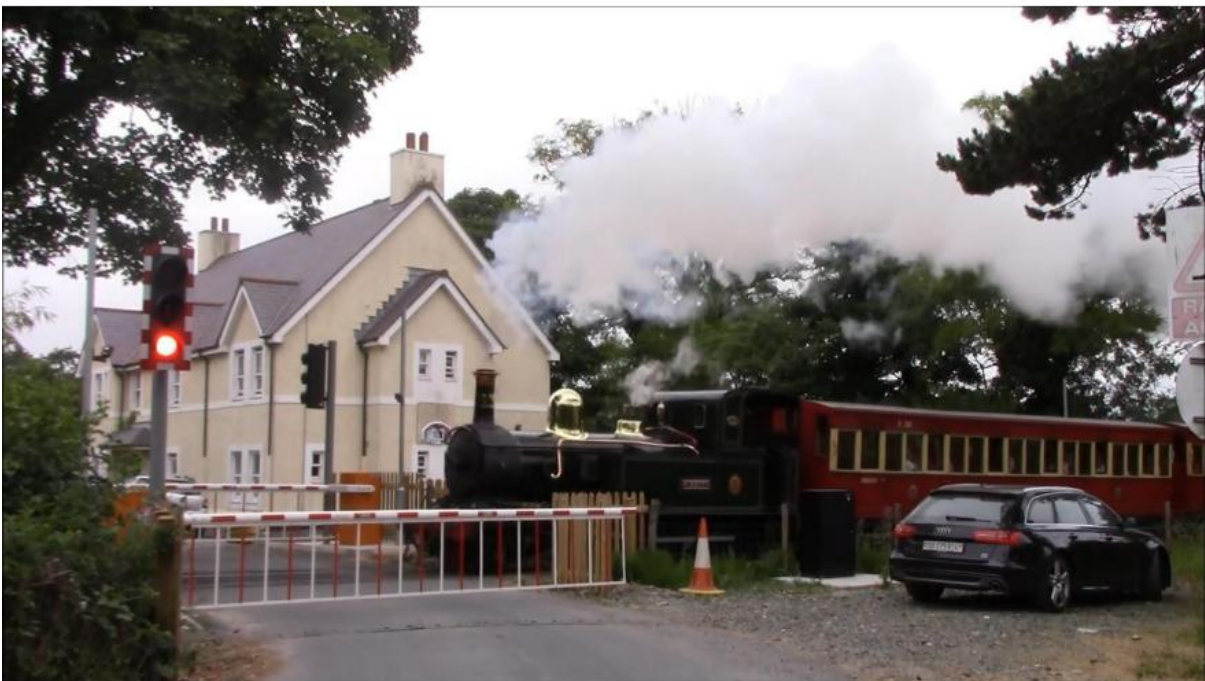
Figure 20 – Simplified Light Rail Barrier Crossing on Isle of Man Steam Railway (Source: YouTube/Perryd Pelle)
