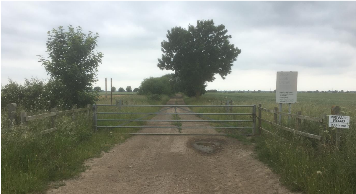
Figure 10 – Typical UWC installation on Wisbech Branch Route (Photo: Alex Dodds)
