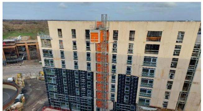
The roof is on, and the internal works have begun with plastering of 7 floors, all bathrooms pods are installed. Brickslip panelling has commenced also. The progress on this site is on track.
