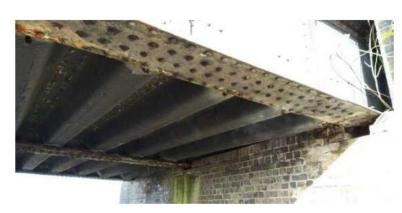
SPALLED BRICKWORK NEAR THE TOP OF ABUTMENT
