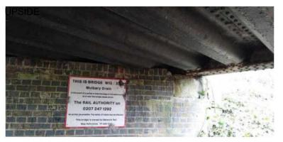
LAMINATED CORROSION OF MAIN GIRDER BOTTOM FLANGE NEAR ABUTMENT
