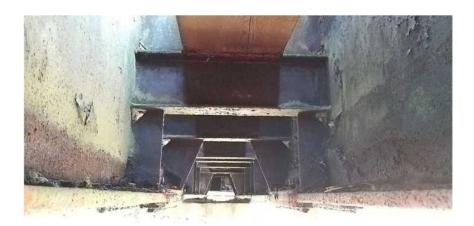
Figure 9 - Chain Bridge - Additional Span - Cross Members
