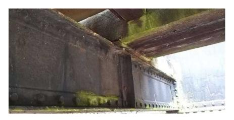
Figure 6 - Chain Bridge - Cross Girder Defects
