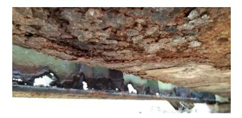
Figure 8 - Chain Bridge - Additional Span - Longitudinal Girder - Bottom Flange Corrosion
