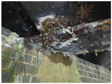
LOSS OF SECTION OF MAIN GIRDER BOTTOM FLANGE **NEAR BEARING**
