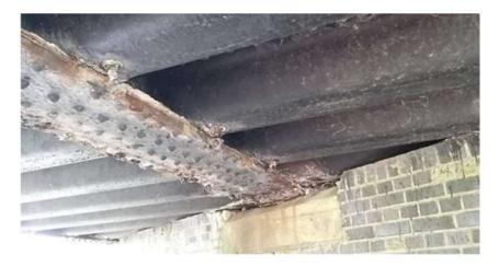
Figure 20 - Lamination & Corrosion - Inner Girder
