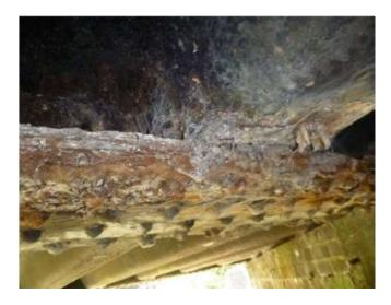
Figure 37 - Redmoor Drain - Outer Girder - Laminated Corrosion
