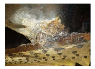
Figure 40 - Redmoor Drain - Transverse Troughing - Corrosion
