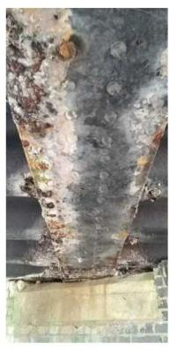
LAMINATION AND PITTING OF MAIN GIRDER BOTTOM FLANGE
