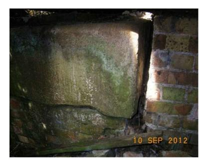
Figure 12 - Chain Bridge - Settlement to High Mileage Abutment
