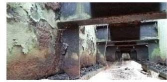
MINOR LAMINATED CORROSION AND PITTING IN STEEL GIRDER
