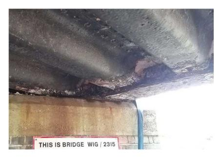
Figure 21 - Lamination & Corrosion - Outer Girder
