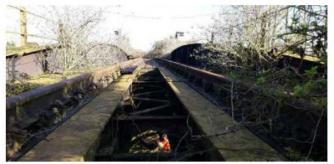
ROTTED / MISSING WAYBEAM AND TIMBER DECK
