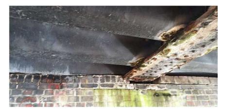
Figure 32 - Waldersey Drain - Transverse Troughing Corrosion
