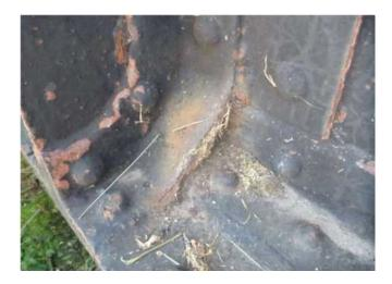
Figure 39 - Redmoor Drain - Transverse Stiffeners - Corrosion
