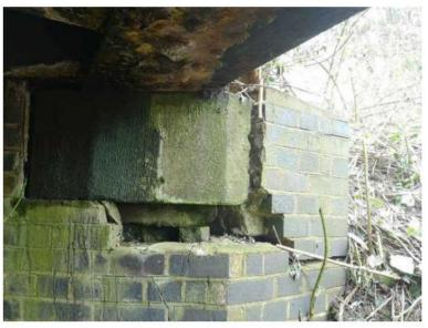
DISLODGED BED STONE AND BRICKWORK AT ABUTMENT CORNER
