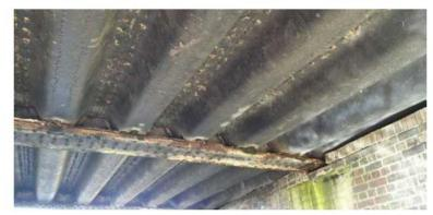
LAMINATED CORROSION OF MAIN GIRDER BOTTOM FLANGE NEAR BEARING
