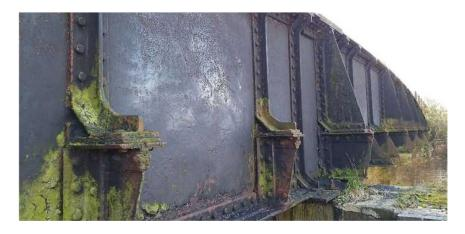
Figure 5 - Chain Bridge - Hog-back Girder - Defects
