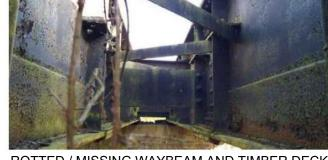
ROTTED / MISSING WAYBEAM AND TIMBER DECK
