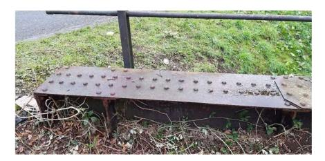
Figure 38 - Redmoor Drain - Topside view of Outer Girder
