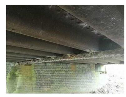
LAMINATED CORROSION OF MAIN GIRDER BOTTOM FLANGE
