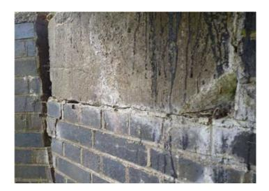
Figure 25 - Low Mileage Abutment Fractured at Bedstone
