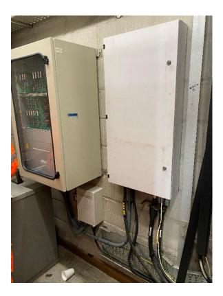
Figure 2: Telephone Concentrator & Telecoms MDF
