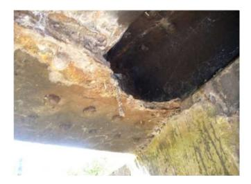
Figure 36 - Redmoor Drain - Low Mileage Outer Girder - Bottom Flange Corrosion
