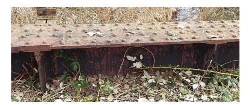
Figure 23 - Typical Condition Top Flange & Web - Outer Girder
