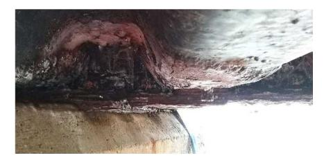
Figure 24 - Localised Trough Corrosion
