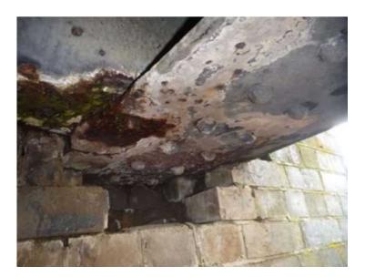
Figure 41 - Redmoor Drain - Abutments - Typical Displaced Brickwork
