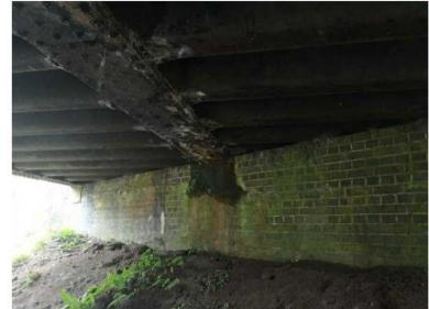
FRACTURED BRICKWORK IN ABUTMENT WALL
