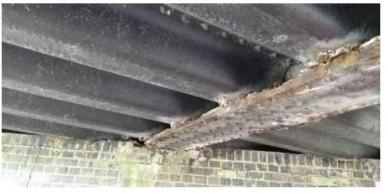
LOSS OF SECTION IN MAIN GIRDER BOTTOM FLANGE NEAR BEARING
