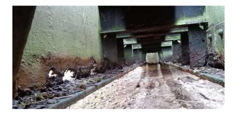
Figure 7 - Chain Bridge - Addition Span - Longitudinal Girder - Web Section Loss
