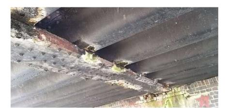
Figure 30 - Waldersey Drain - Inner Girder - Bottom Flange Corrosion
