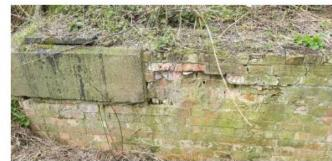
FRACTURED AND DISPLACED ABUTMENT
