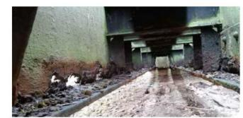
LOSS OF SECTION IN MAIN GIRDER WEB NEAR BOTTOM FLANGE
