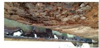
LAMINATED CORROSION IN MAIN GIRDER BOTTOM FLANGE
