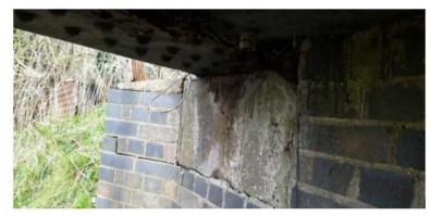
FRACTURED BED STONE AND BRICKWORK AT ABUTMENT CORNER
