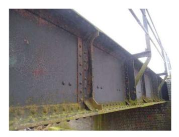
Figure 31 - Outer Girder - Surface Corrosion
