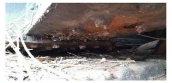
LOCALISED CORROSION IN MAIN GIRDER BOTTOM FLANGE NEAR BEARING
